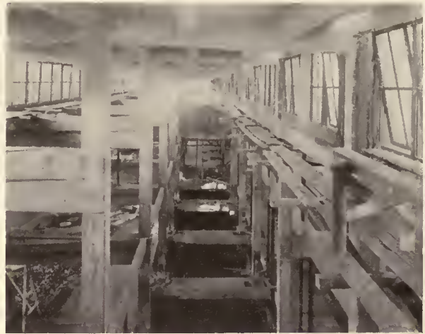
MONITOR OPEN OVENS Showing special construction in floors below
